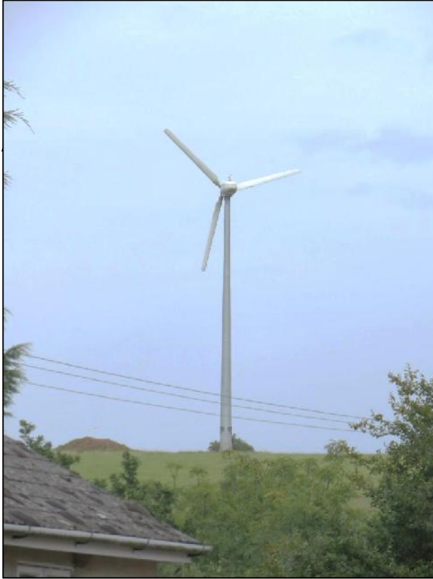
Figure 3.1: 'Small' wind turbine (27m) found in Teignbridge district
